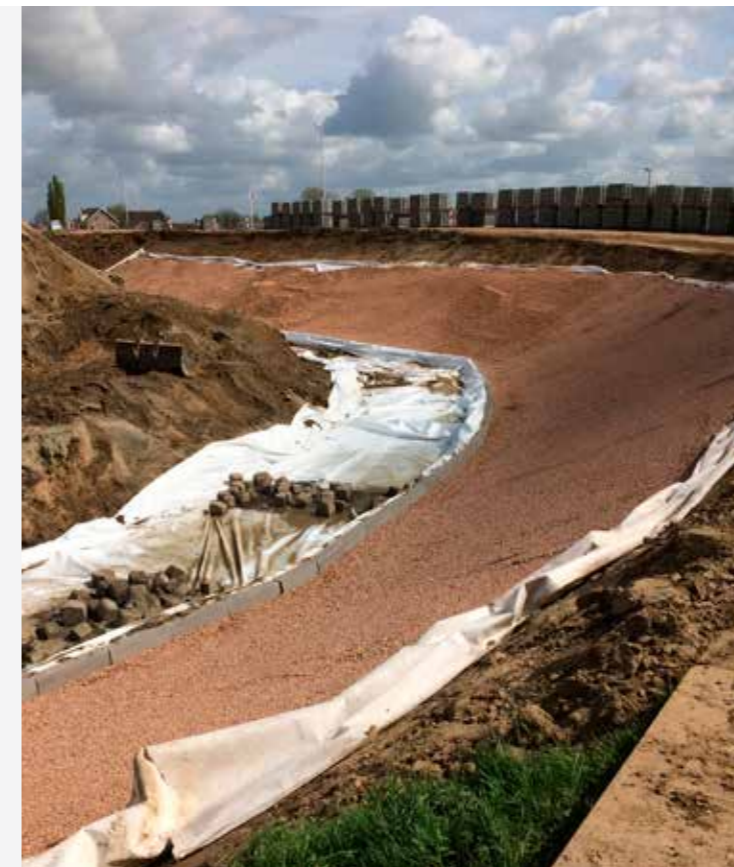
Bontec NW Geotextiles used in dyke constructions will prevent the movement of soil particles (piping). Piping is the phenomenon of soil particles being transported by seeping water, creating tubular openings under the dyke.
