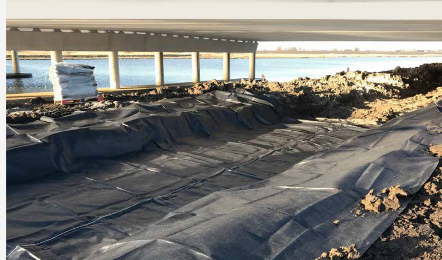
Bontec SG In the foundation of new road constructions geotextiles are used for separation and filtration purposes to prevent granular material being mixed. This increases the lifetime of roads.
