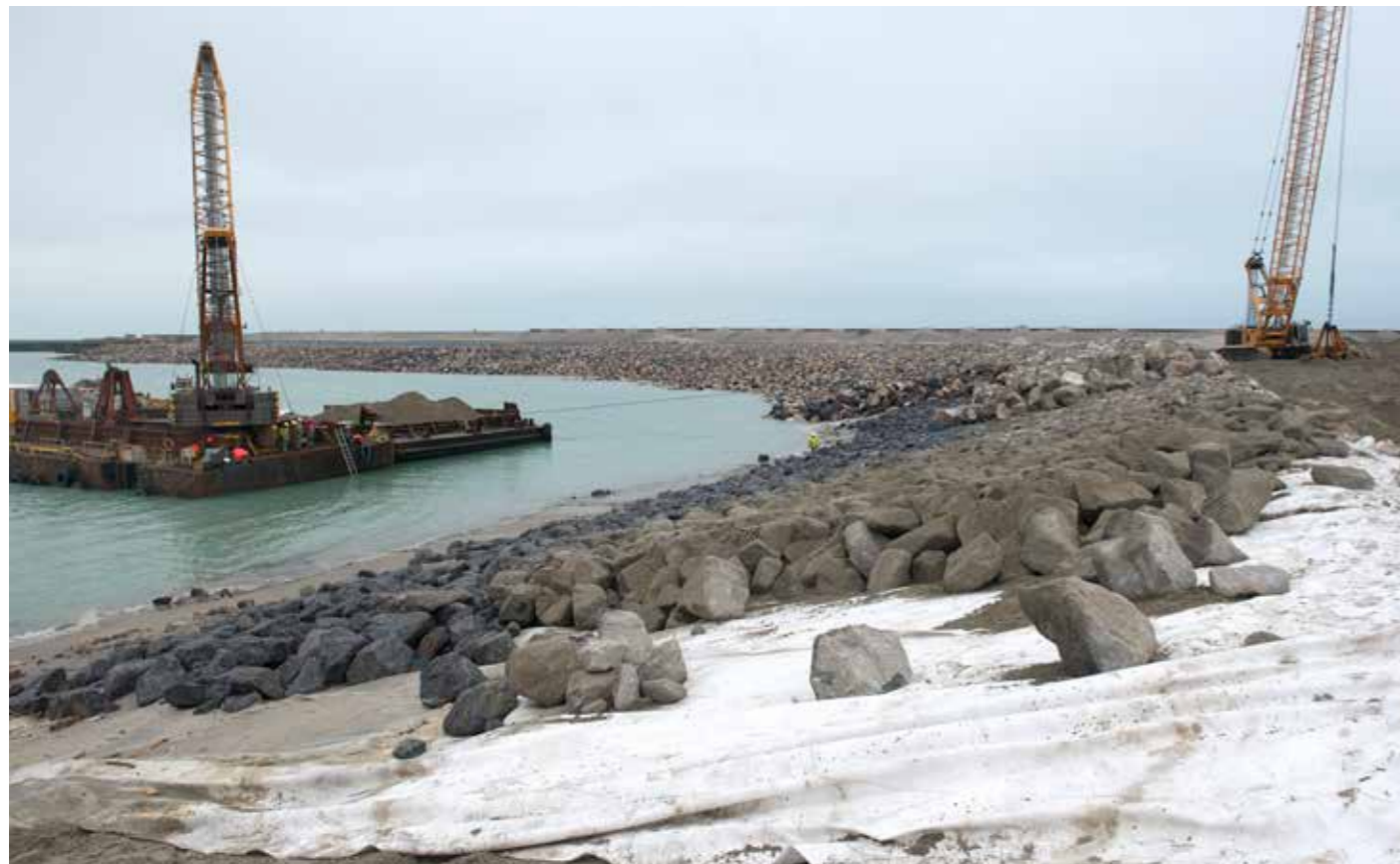
Bontec Protec Traditional rock revetments are build up from fine to coarse granules to form a natural filter. The use of geotextiles can replace up to 1 m of this natural filter, whilst preventing any possible wash-out of sand.
