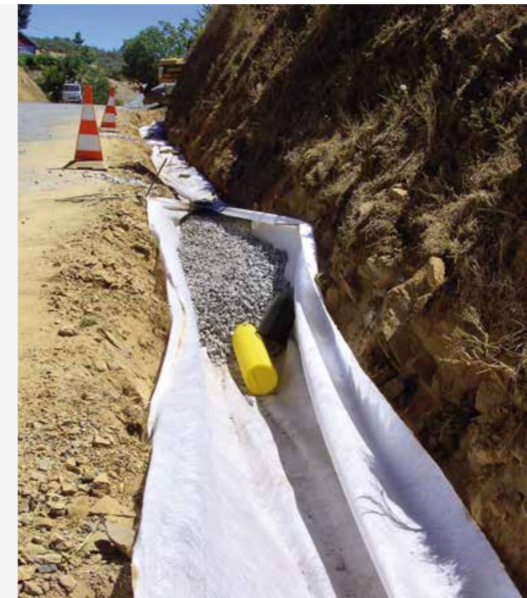
Bontec NW Wrapped around French drains Bontec will act as a filter layer, reducing the need for granular fill and preventing the backfill from silting up.
